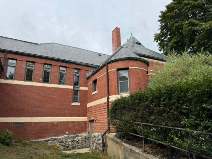
Fig. 8. Exposed granite rubble foundation wall on east elevation.
