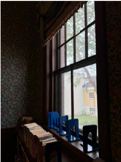
Fig. 11. Original double hung wood window.
