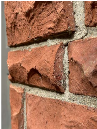
Fig. 5. Cut rusticated base showing clay or cement and aggregate matrix.
