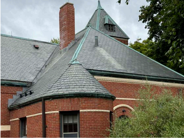
Fig. 10. Copper gutters, downspouts, valleys and hips.
