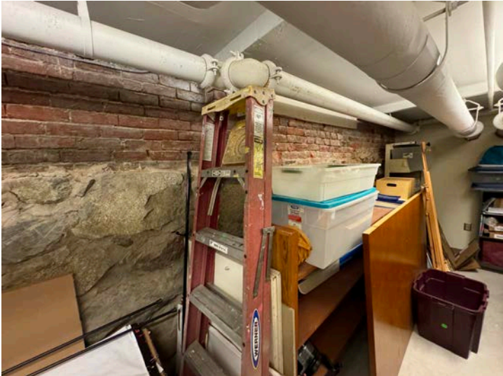
Fig. 24. Basement walls – brick and rubble stone.
