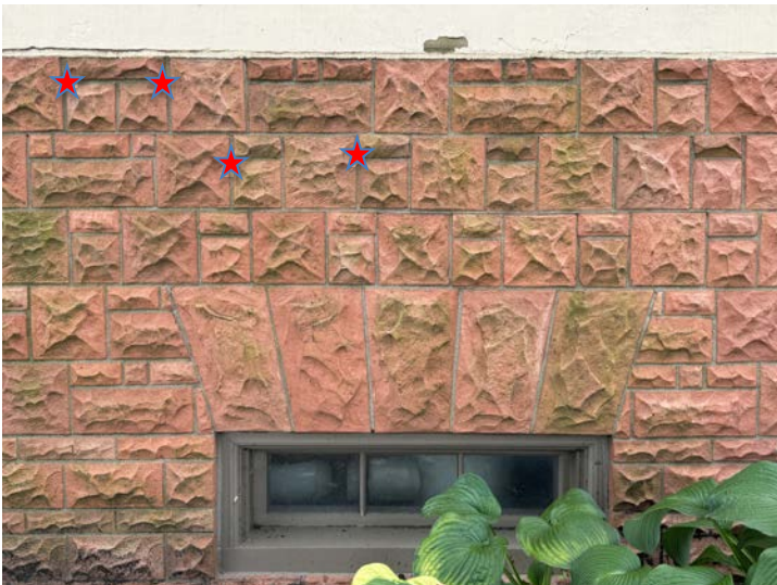
Fig. 6. Rusticated base showing duplicate cast patterns.
